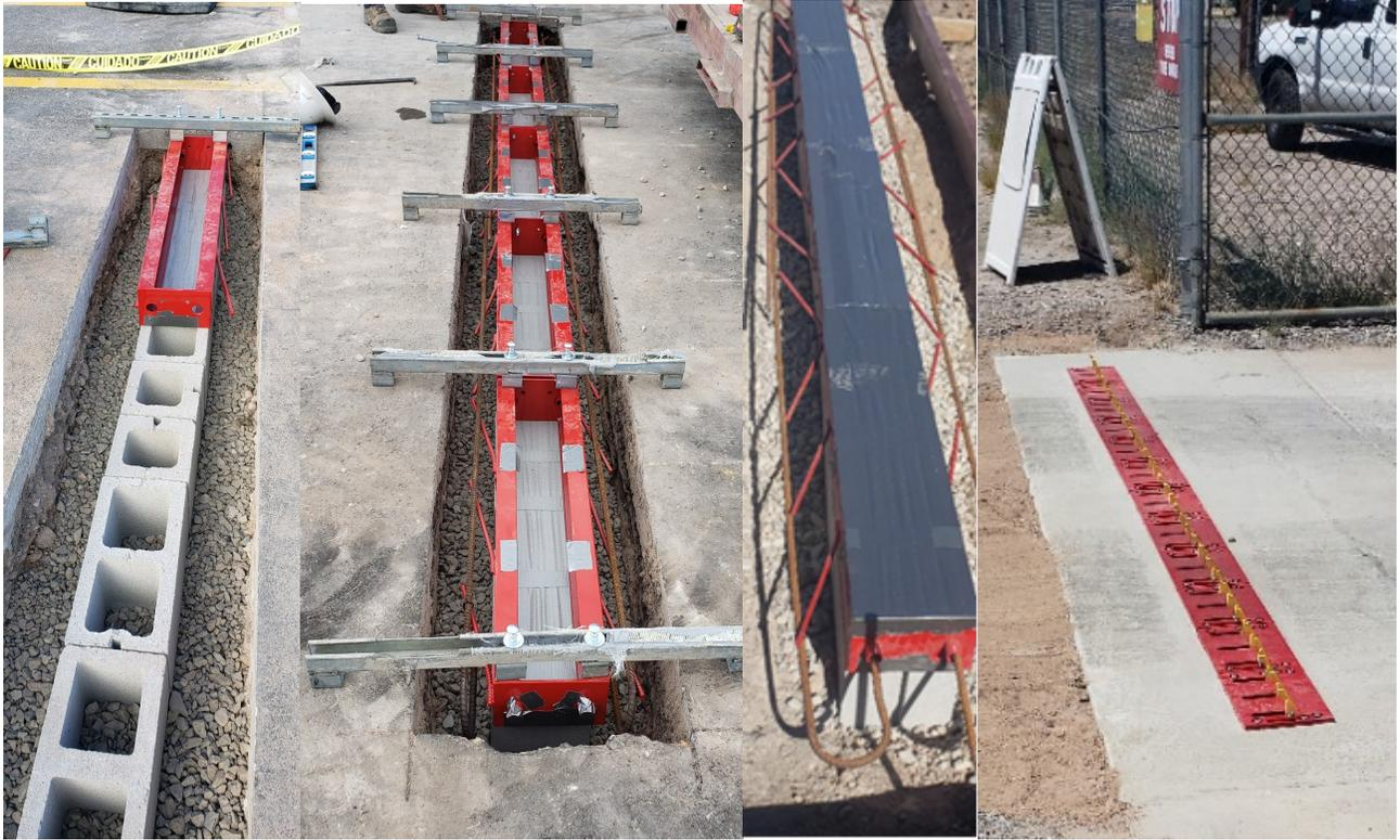
1. Excavate the placement area 24 to 48 inches deep (depending on drainage needs in your area) by at least 12" longer and 8" wider than the units you are installing.
